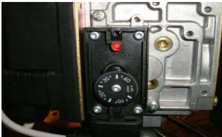
Fig 7.3.2 - Low Gas Inlet Pressure Switch
